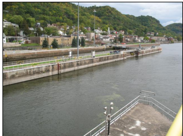
Lock is 110 ft wide by 600 ft long
