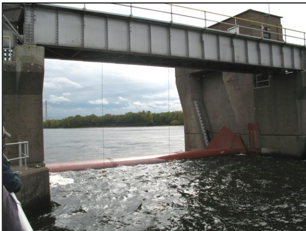
Roller gate dam section
