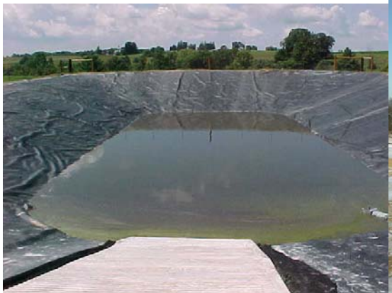
Plastic Lined Storage Pond
