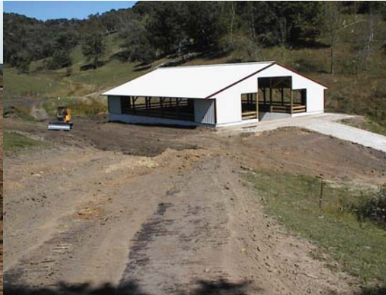
Roofed Storage Structure
