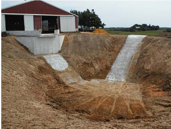
Earthen Storage Facility
